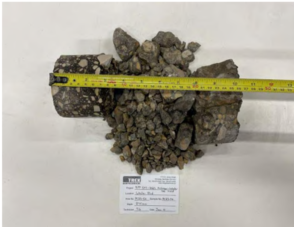
Photo 56: Pavement Core Sample PC23-56
