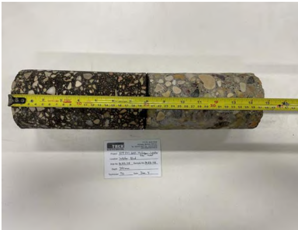
Photo 48: Pavement Core Sample PC23-48
