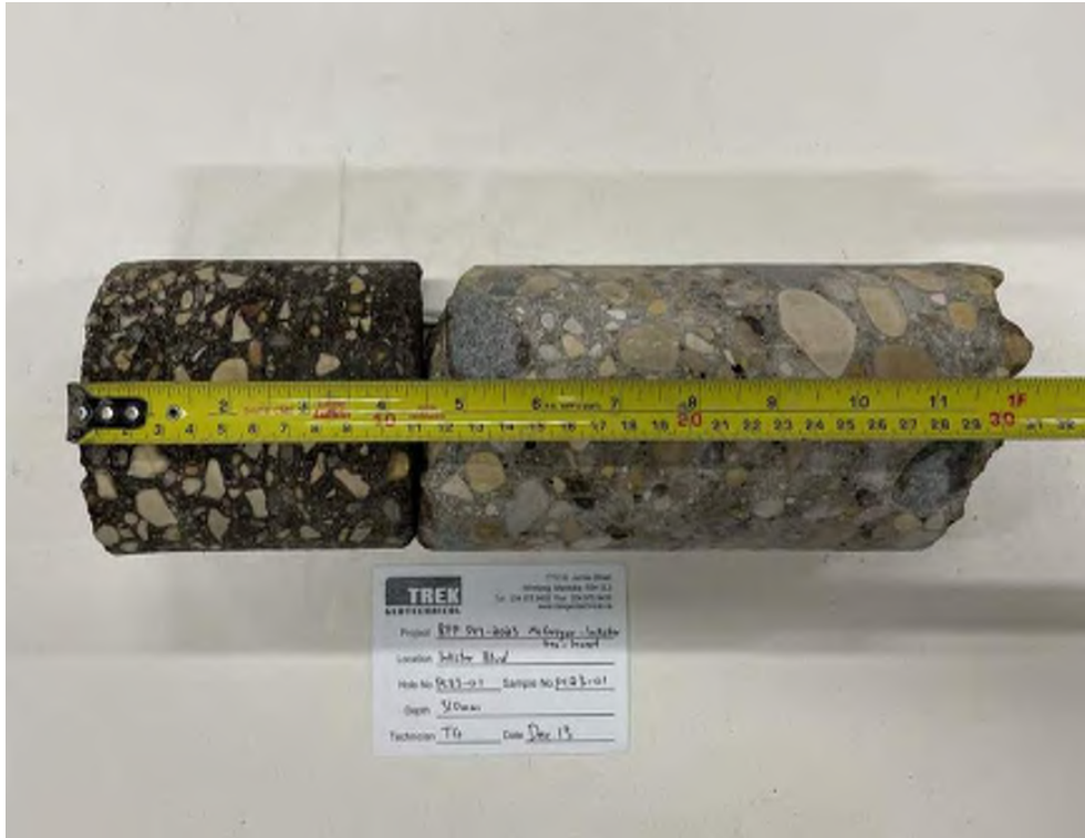
Photo 1: Pavement Core Sample PC23-01
