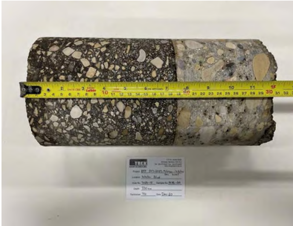
Photo 5: Pavement Core Sample at Test Hole TH23-15
