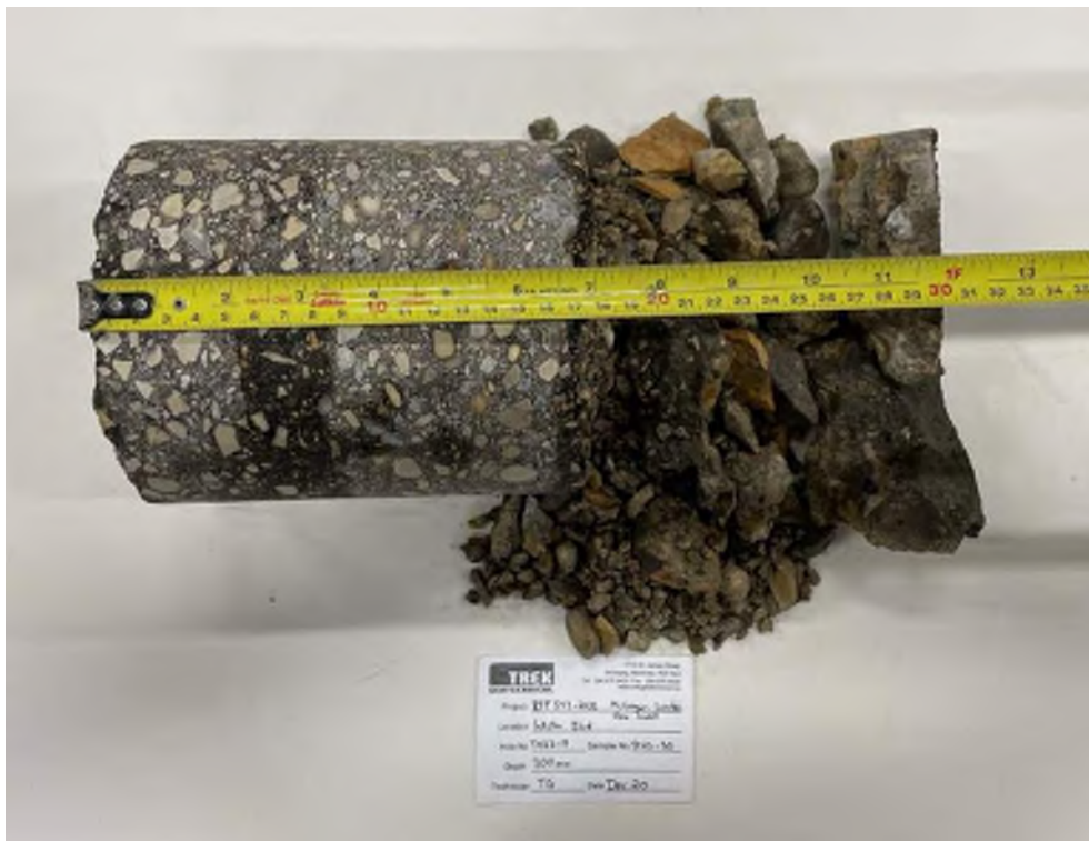
Photo 30: Pavement Core Sample PC23-30
