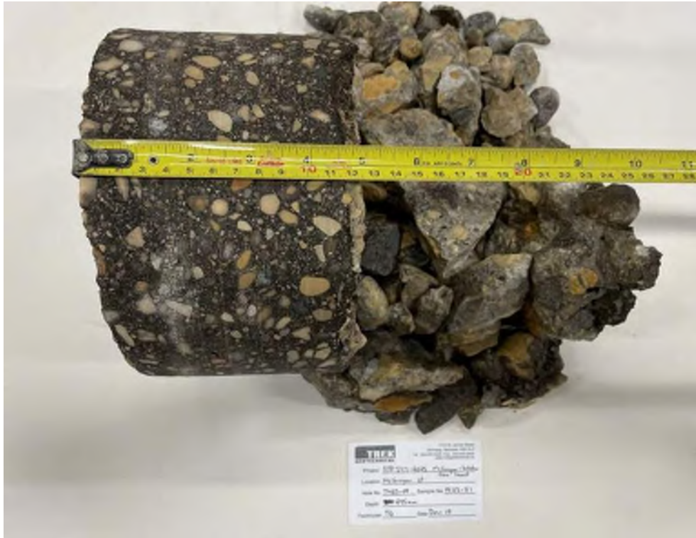
Photo 9: Pavement Core Sample at Test Hole TH23-09
