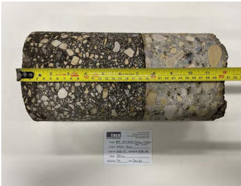
Photo 26: Pavement Core Sample PC23-26
