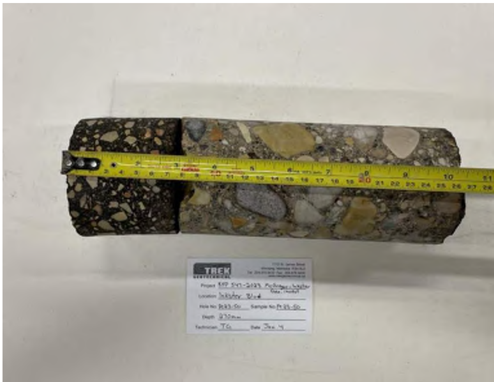
Photo 50: Pavement Core Sample PC23-50
