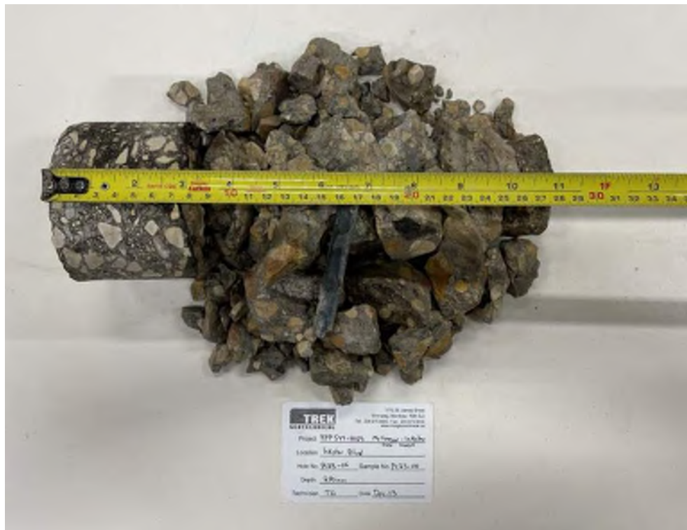
Photo 6: Pavement Core Sample PC23-06
