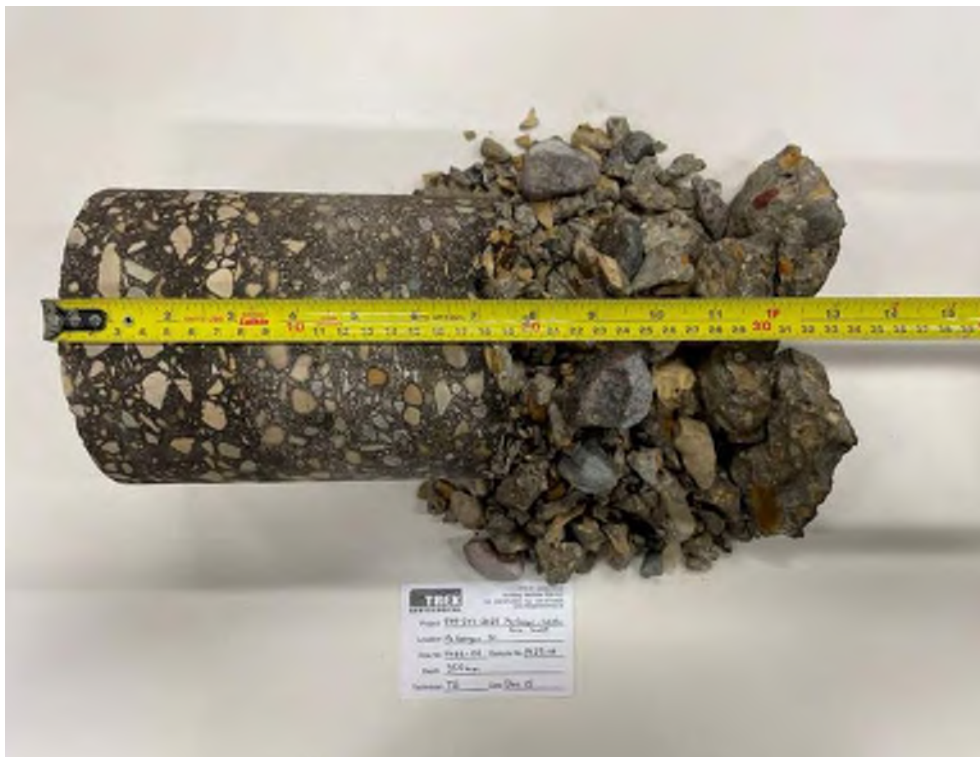
Photo 6: Pavement Core Sample at Test Hole TH23-06
