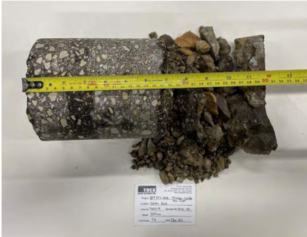
Photo 9: Pavement Core Sample at Test Hole TH23-19
