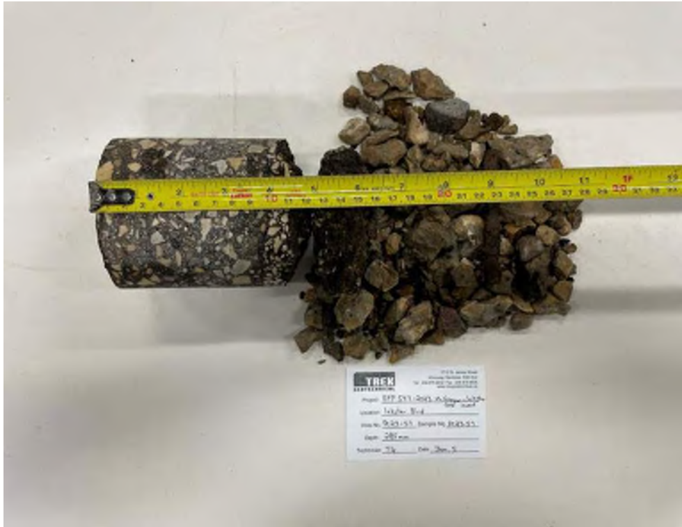
Photo 57: Pavement Core Sample PC23-57
