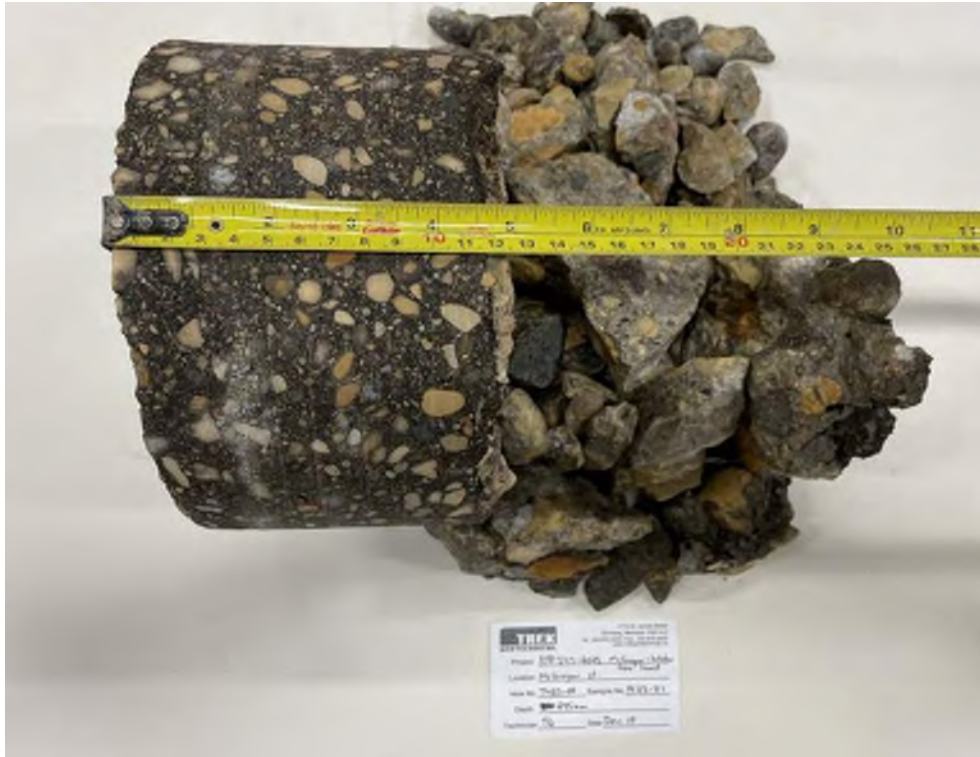
Photo 21: Pavement Core Sample PC23-21
