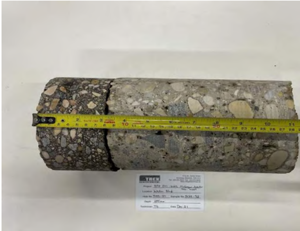
Photo 1: Pavement Core Sample at Test Hole TH23-21
