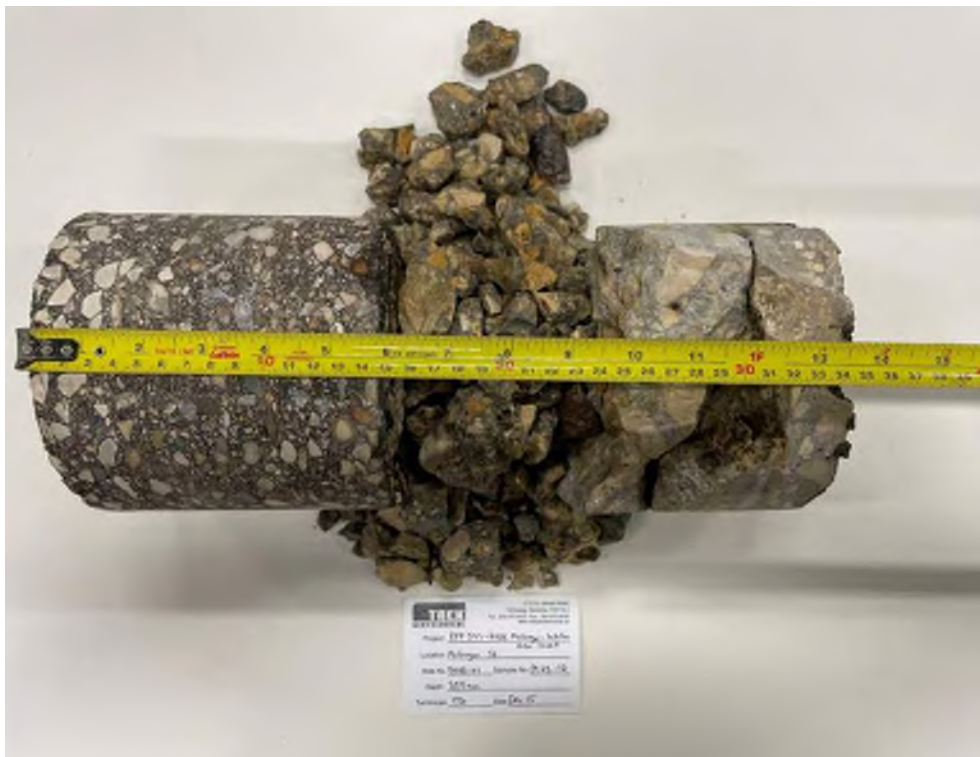
Photo 12: Pavement Core Sample PC23-12
