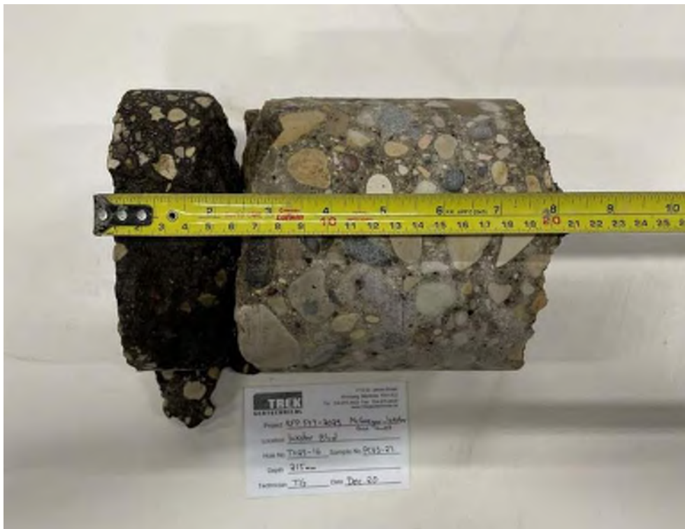
Photo 6: Pavement Core Sample at Test Hole TH23-16
