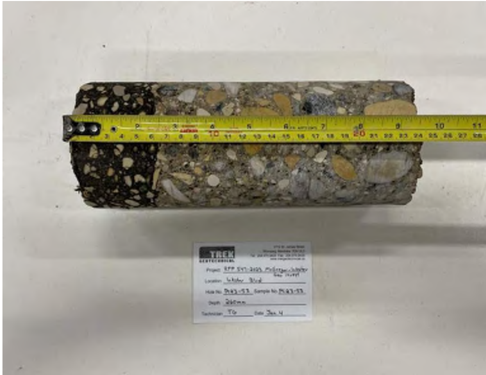
Photo 53: Pavement Core Sample PC23-53
