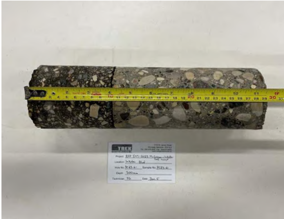
Photo 61: Pavement Core Sample PC23-61
