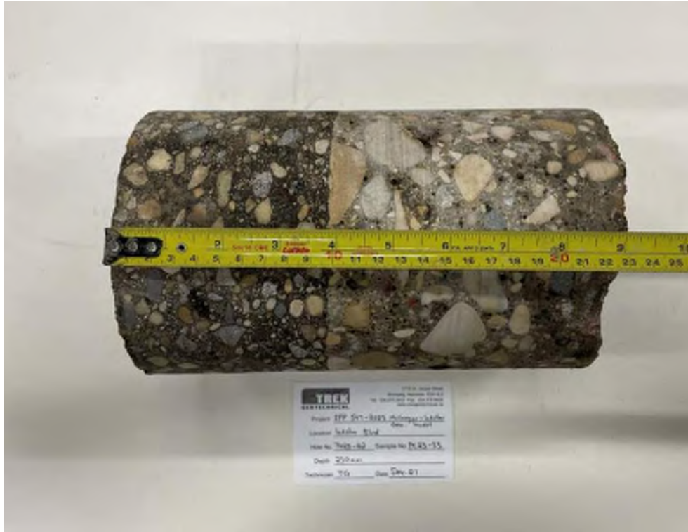
Photo 33: Pavement Core Sample PC23-33
