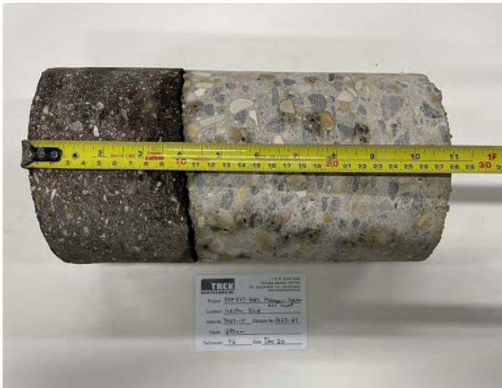
Photo 4: Pavement Core Sample at Test Hole TH23-14
