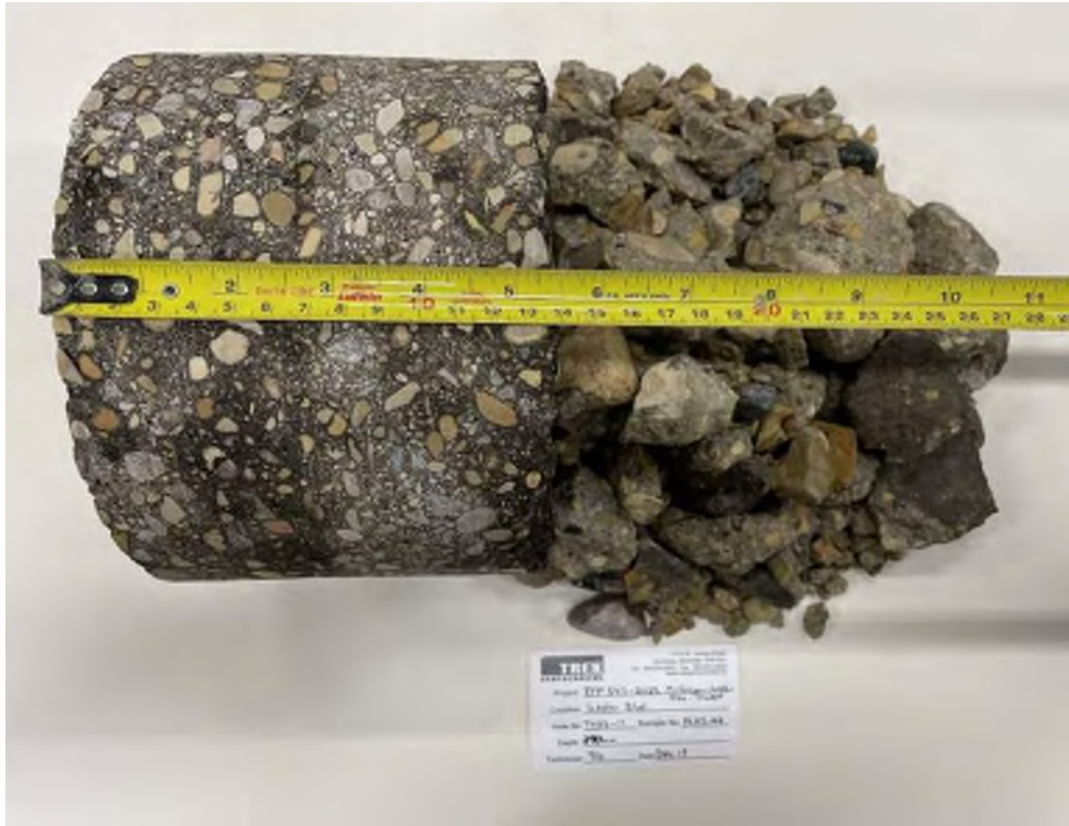
Photo 1: Pavement Core Sample at Test Hole TH23-11
