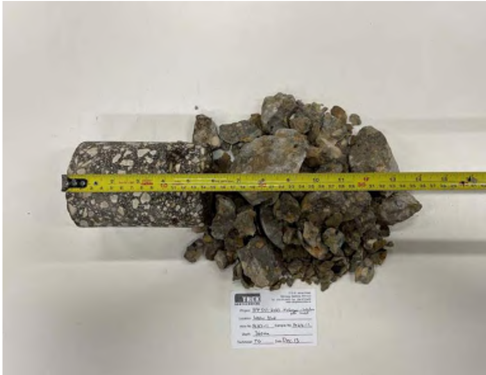
Photo 11: Pavement Core Sample PC23-11
