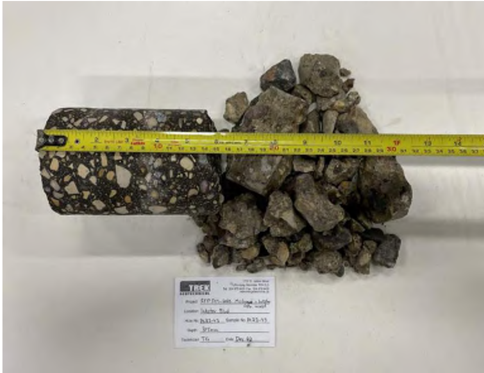
Photo 43: Pavement Core Sample PC23-43
