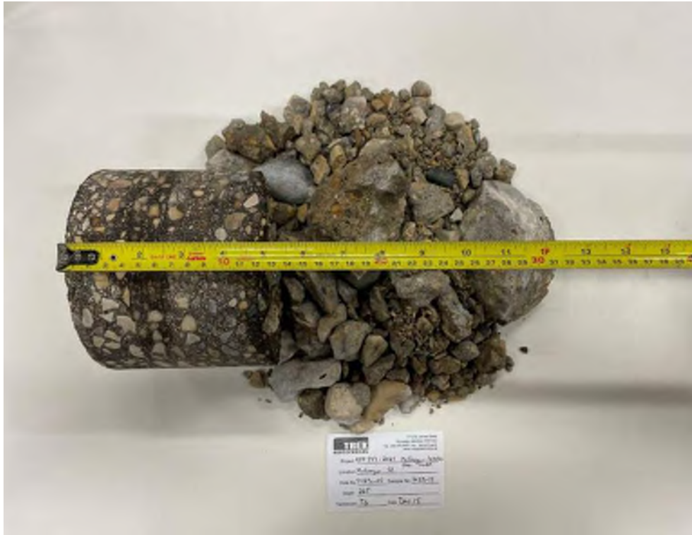
Photo 15: Pavement Core Sample PC23-15
