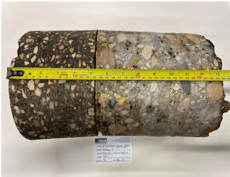
Photo 4: Pavement Core Sample at Test Hole TH23-04
