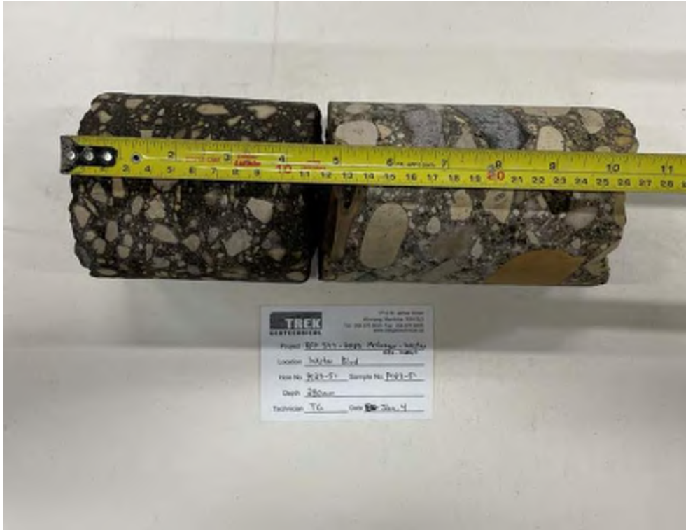
Photo 51: Pavement Core Sample PC23-51
