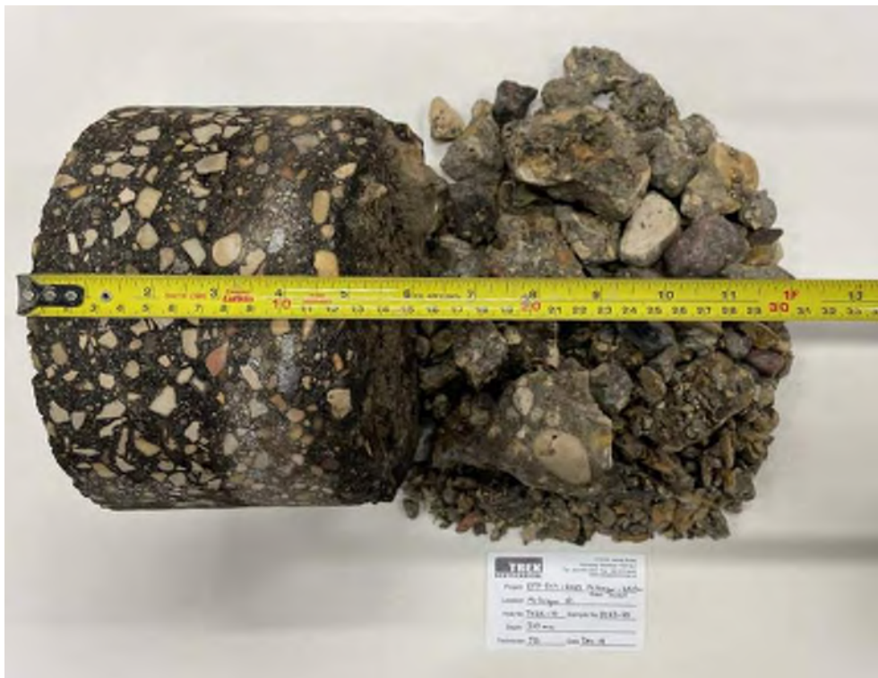
Photo 20: Pavement Core Sample PC23-20
