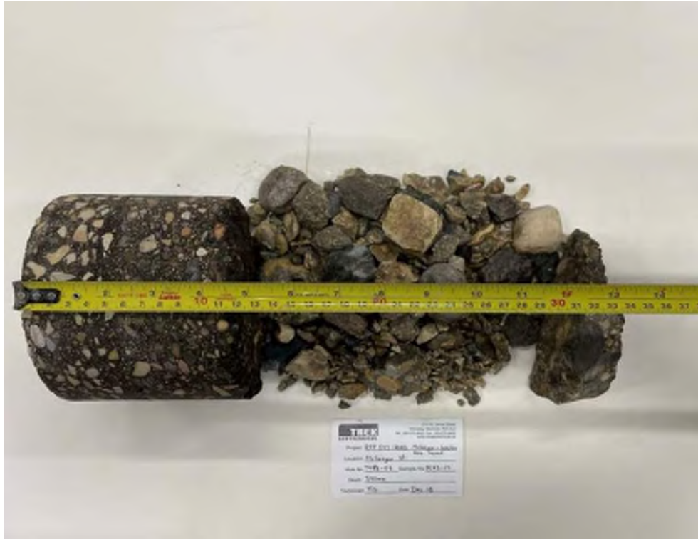
Photo 3: Pavement Core Sample at Test Hole TH23-03
