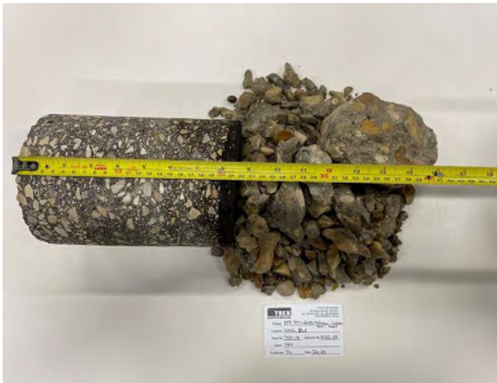
Photo 8: Pavement Core Sample at Test Hole TH23-18
