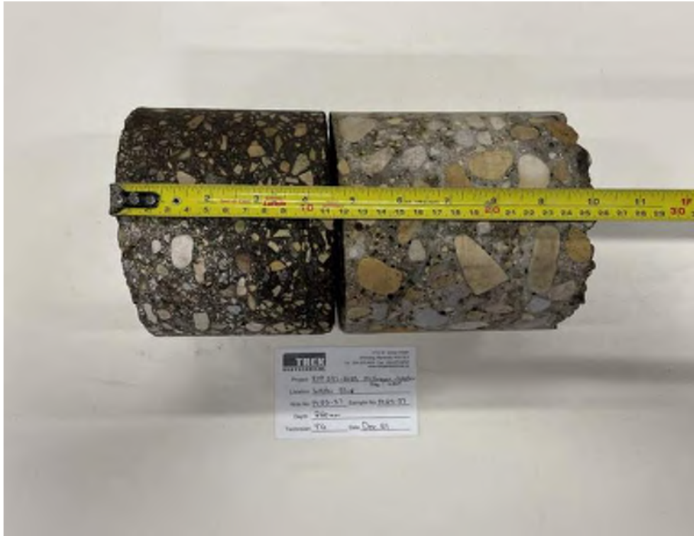
Photo 37: Pavement Core Sample PC23-37
