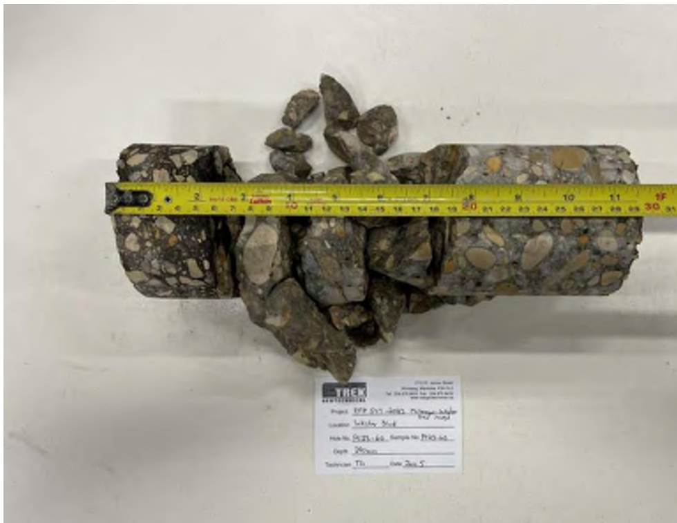
Photo 60: Pavement Core Sample PC23-60
