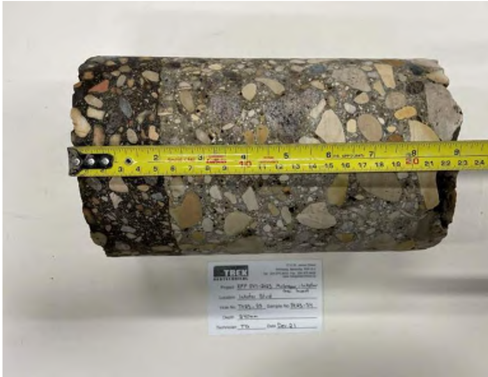
Photo 3: Pavement Core Sample at Test Hole TH23-23
