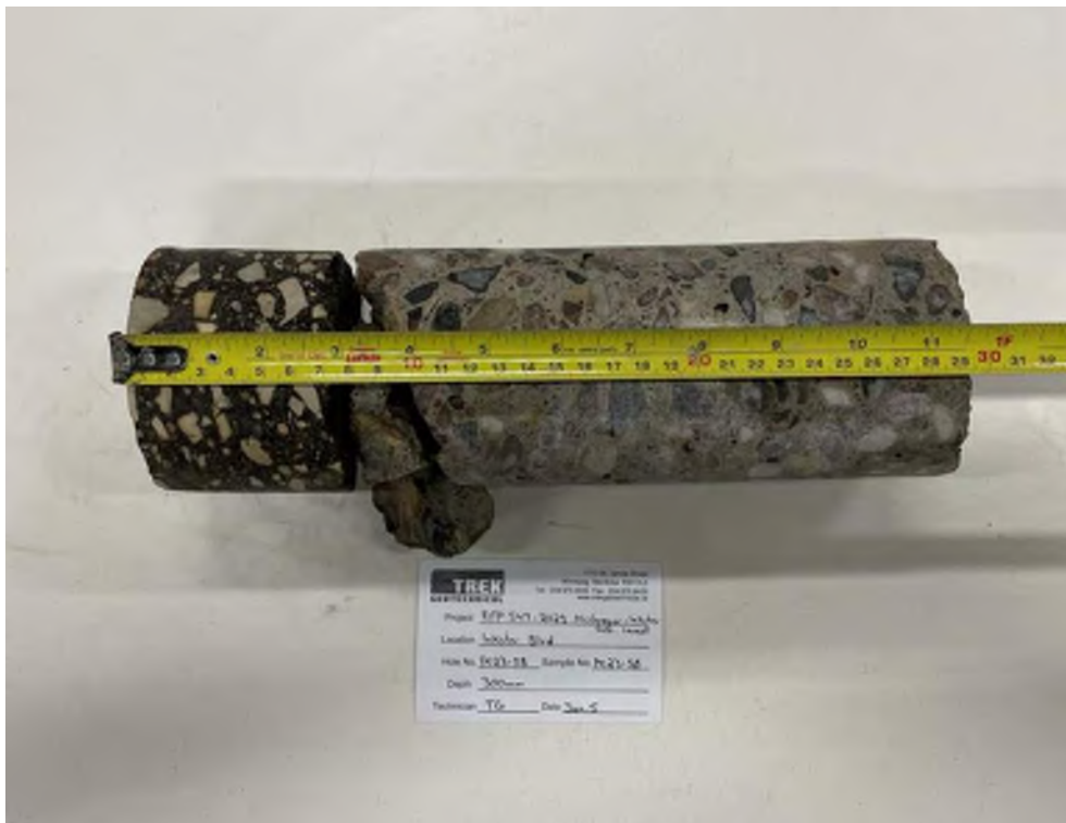
Photo 58: Pavement Core Sample PC23-58
