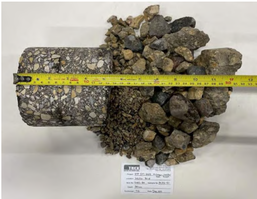
Photo 10: Pavement Core Sample at Test Hole TH23-20
