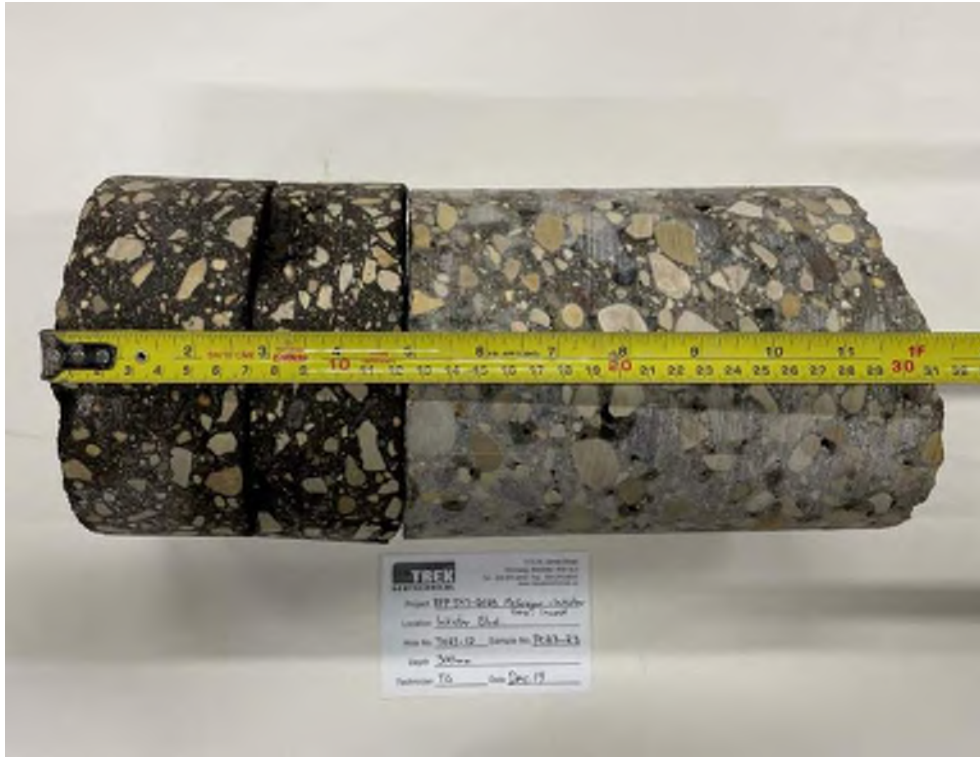
Photo 23: Pavement Core Sample PC23-23
