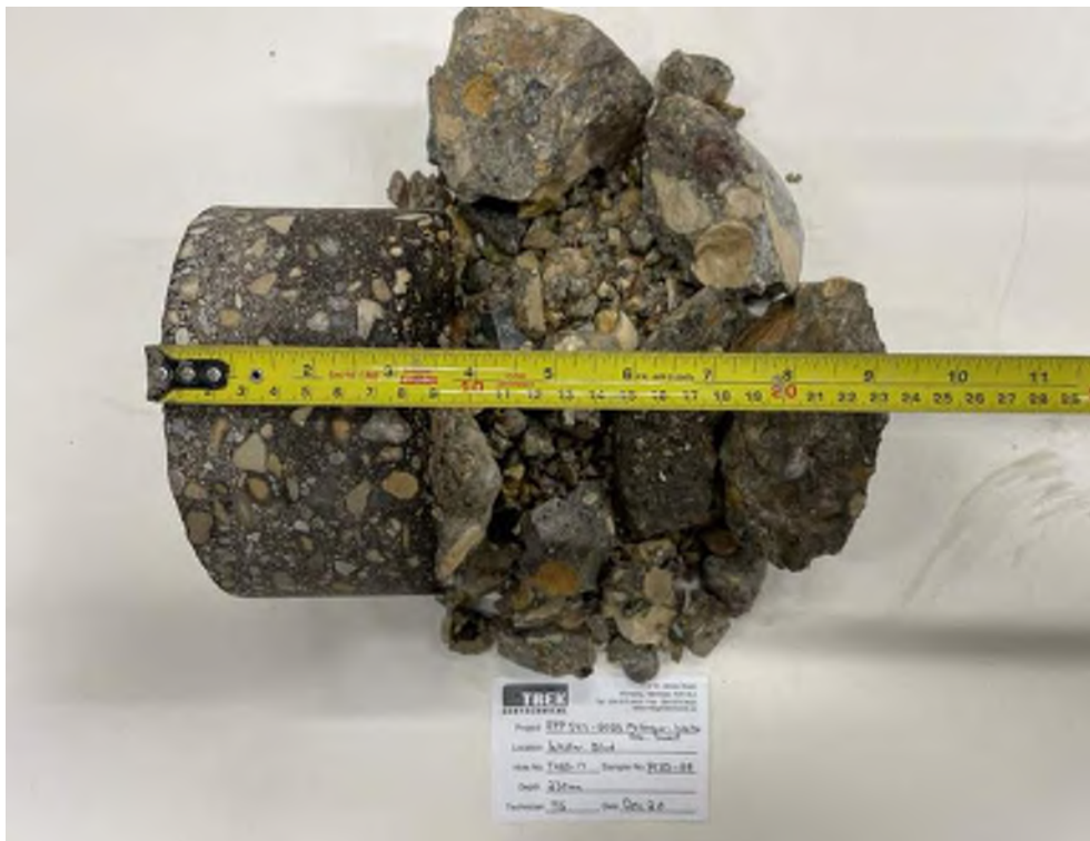
Photo 28: Pavement Core Sample PC23-28
