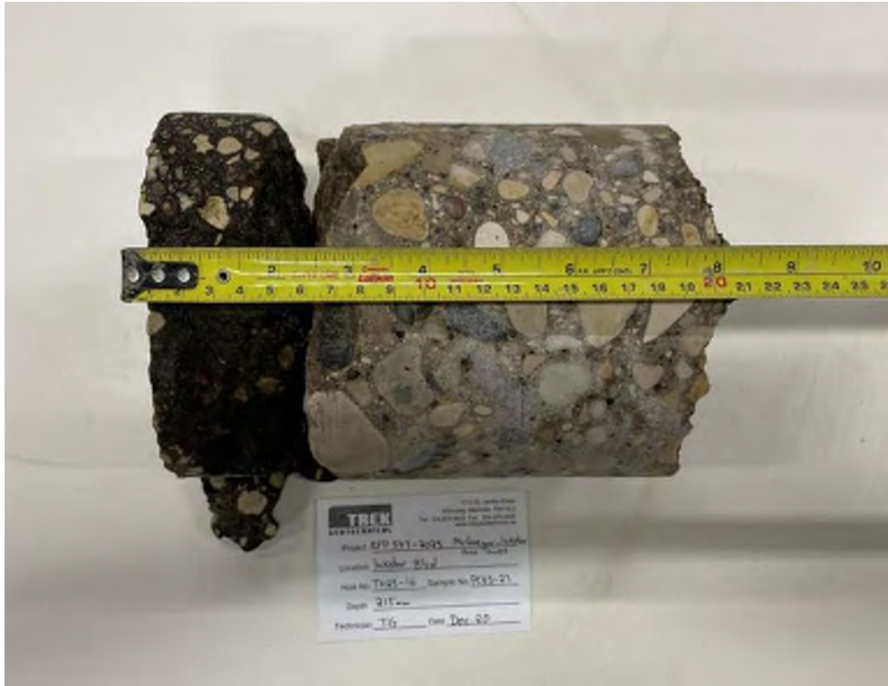
Photo 27: Pavement Core Sample PC23-27
