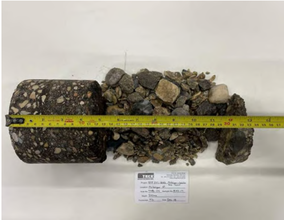
Photo 17: Pavement Core Sample PC23-17
