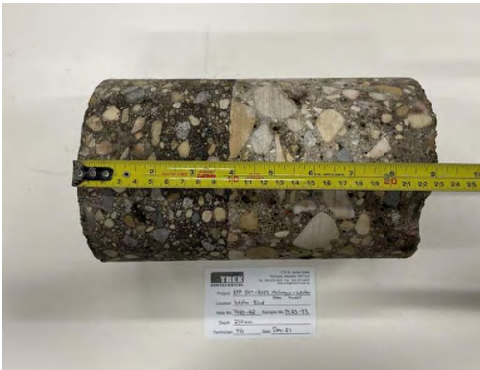
Photo 2: Pavement Core Sample at Test Hole TH23-22
