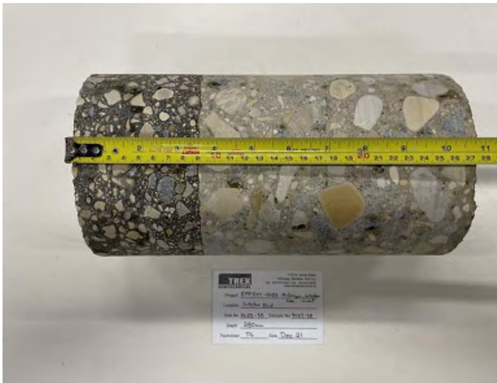
Photo 38: Pavement Core Sample PC23-38
