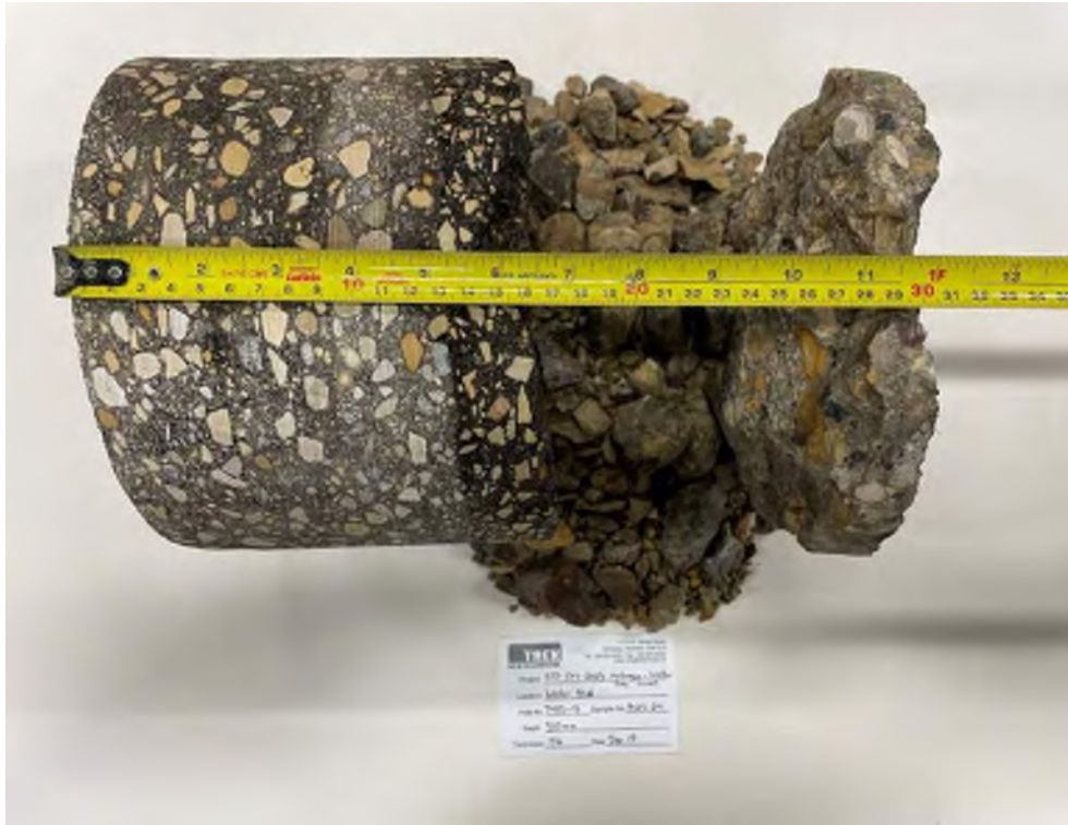
Photo 3: Pavement Core Sample at Test Hole TH23-13
