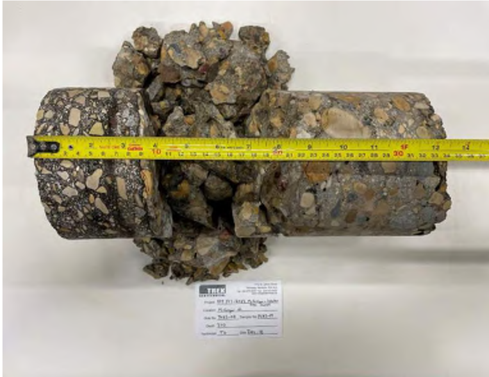
Photo 19: Pavement Core Sample PC23-19
