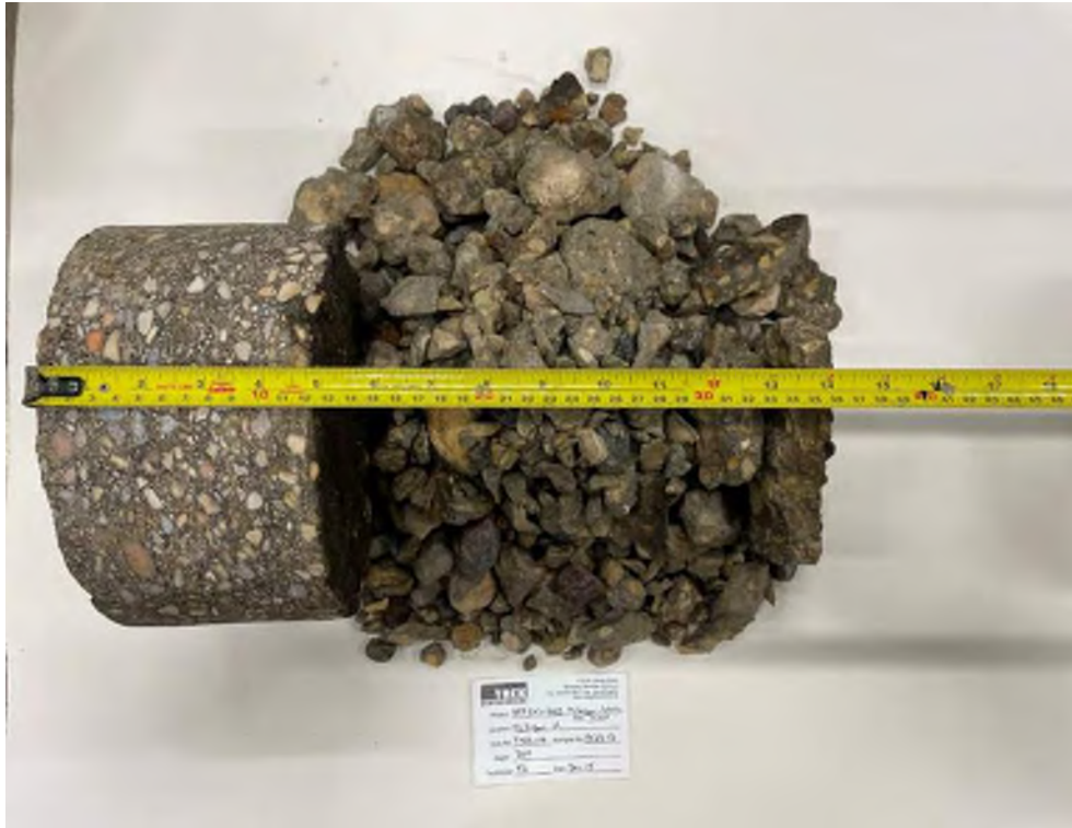
Photo 13: Pavement Core Sample PC23-13
