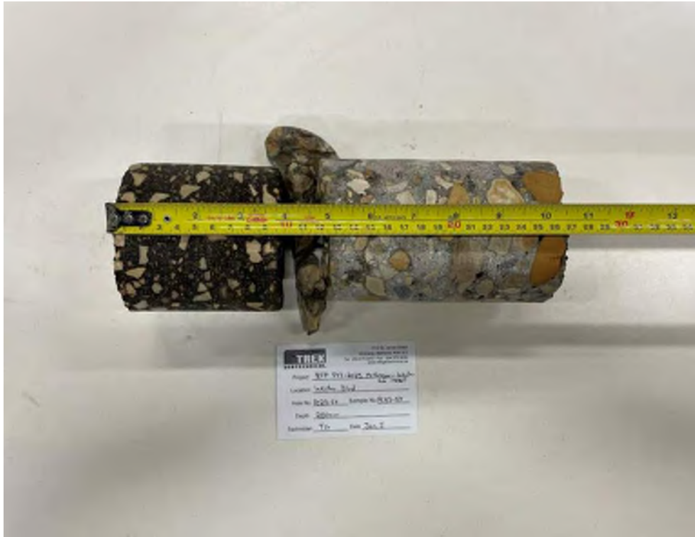
Photo 59: Pavement Core Sample PC23-59
