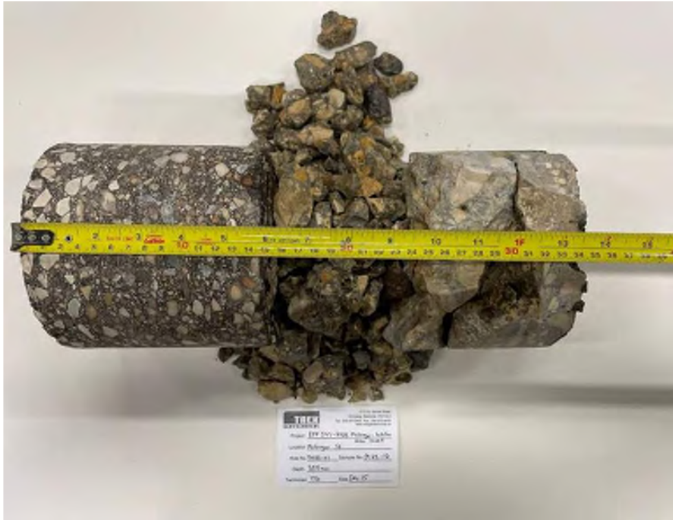
Photo 1: Pavement Core Sample at Test Hole TH23-01
