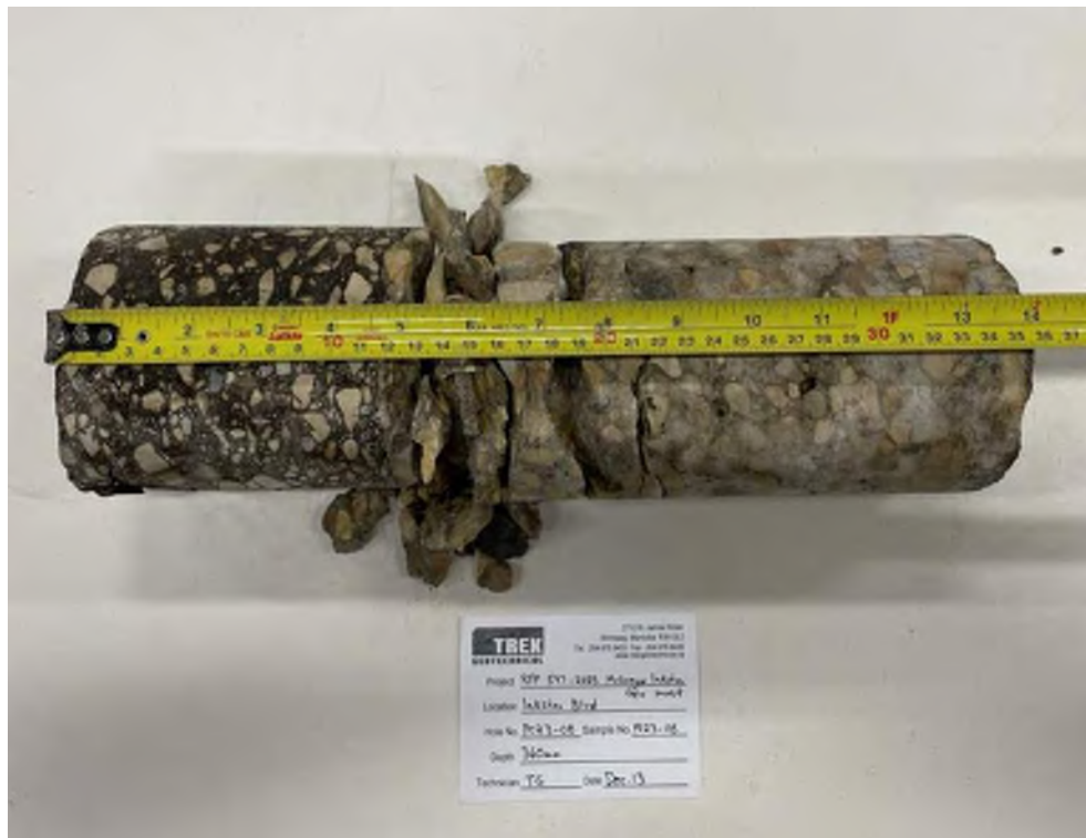
Photo 8: Pavement Core Sample PC23-08
