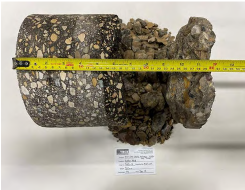
Photo 24: Pavement Core Sample PC23-24
