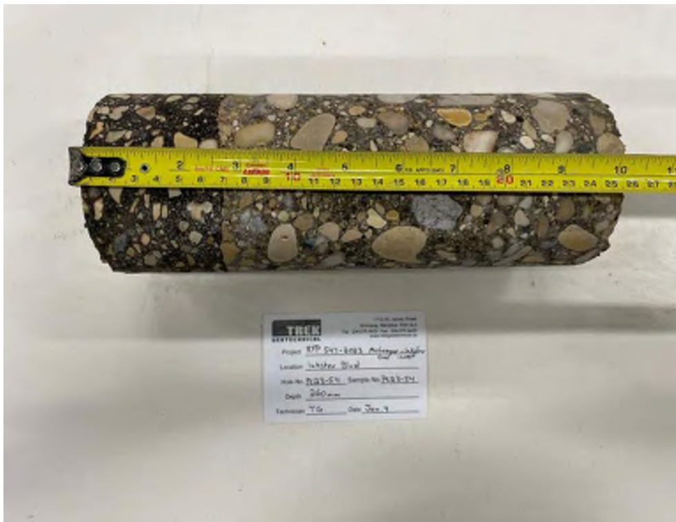
Photo 54: Pavement Core Sample PC23-54
