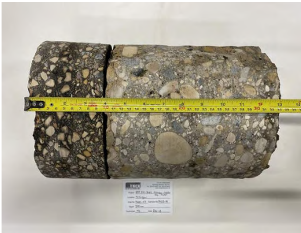
Photo 18: Pavement Core Sample PC23-18
