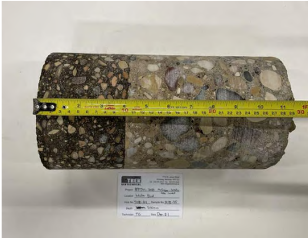
Photo 35: Pavement Core Sample PC23-35
